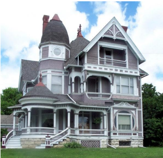
James A. Beck House. Fairfield, Iowa, EUA Fonte: isarchitecture.com
